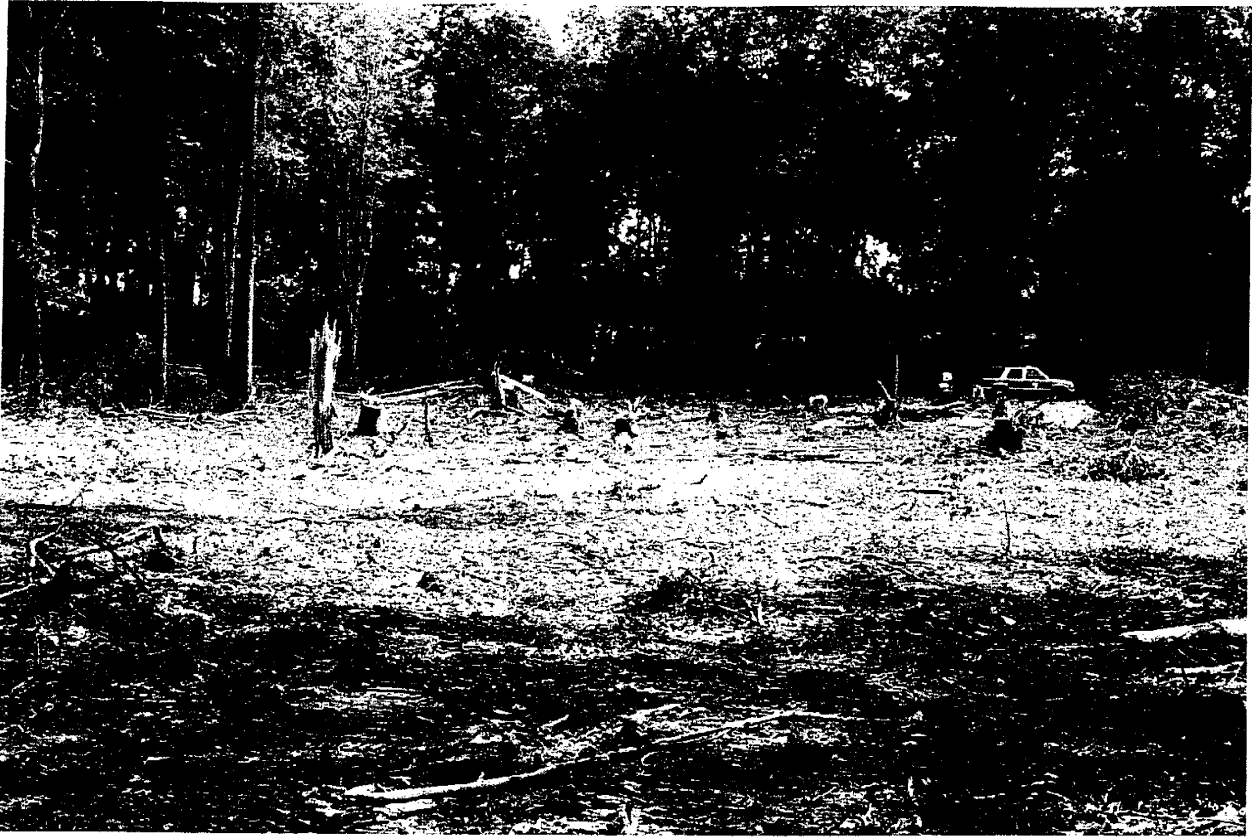
View from back of lot out toward Trundle Road showing cleared area. Note 555 Tracked Loader marks in near foreground.
